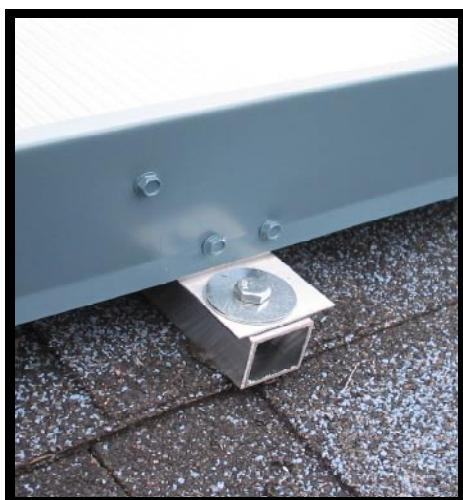
**Position the Ell bracket between the trim and frame so it is CENTERED over the Lag hole.** Install the collector onto the rails with the mounting bracket tab UNDER the trim and BETWEEN the frame. The small bend at the bottom of the trim makes inserting the mounting bracket easy. Be sure to press the collector all the way down on the mounting rail and secure with two 1/4" color coded self tap screws evenly just above the small bend in the trim. **Be sure to catch the tab with both screws!**
